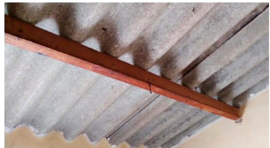
Asbestos-containing ceiling.
